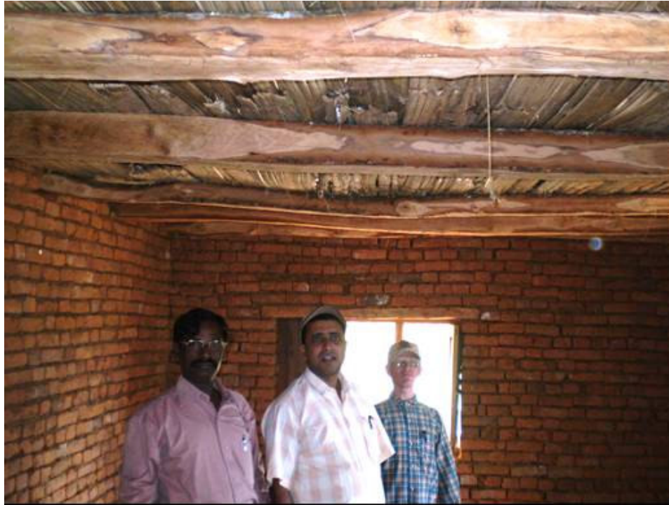
Figure 5: False roof made with bamboos clay in the improved rearing house for providing a cool & comfort atmosphere for rearing purpose
