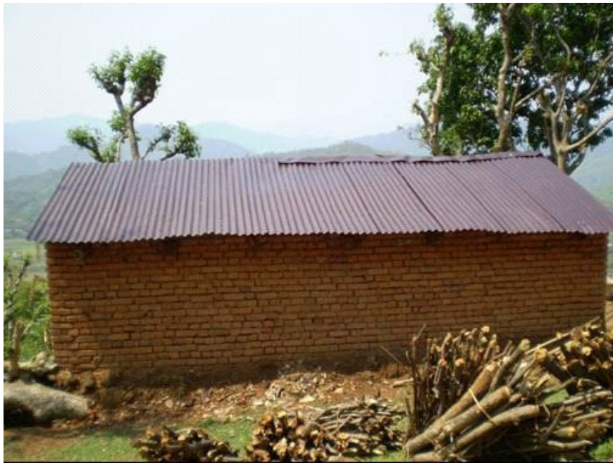
Figure 3: A view of the improved rearing house with G.I roof
